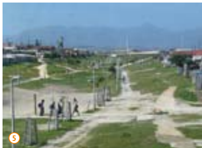
Figure 97 Some parts of the cycle path are situated in a depression, thus further compromising the safety of cyclists and pedestrians
